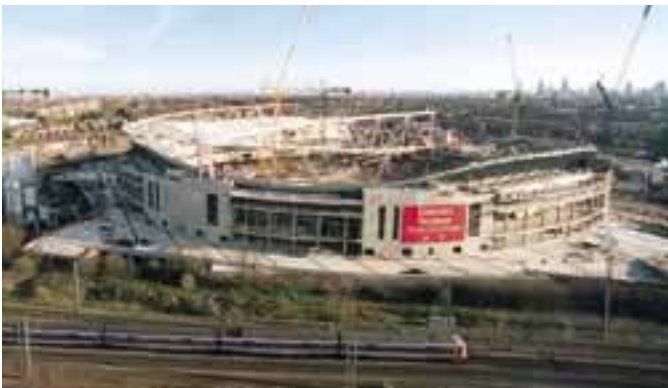
Das Emirates Stadium in London
